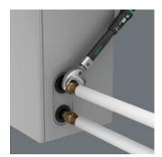
With the 9530 set, the screw connections used for refrigeration and air conditioning systems as well as heat pump lines can be properly tightened.
