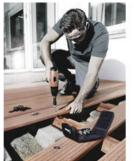
Bit holder for evenly flush countersunk screws in patio construction
